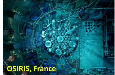
Most common design of research reactors, called the pool type, has a core (fuel elements and control rods) immersed in an open pool of water; the layer of water directly above the reactor core shields the radiation so completely that operators may work close to the reactor safely.
